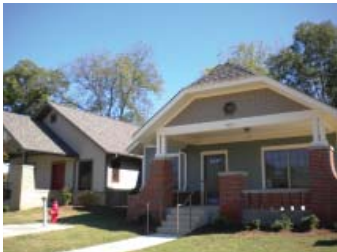
High quality construction and design in affordable housing development by the YWCA sets a desirable standard for future housing investments in the area.
