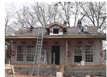
New home under construction by Birmingham Affordable Rental Community on 2nd Court North
