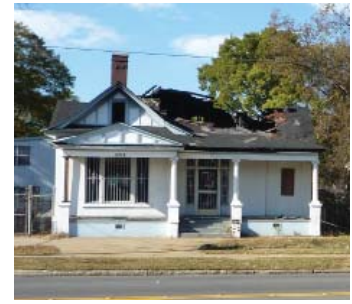
Dilapidated buildings along one of Woodlawn’s primary roads have a significant impact on the community’s image.
